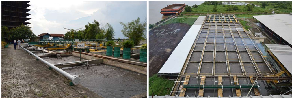
Figure 1 WWTP No.1 (left) and No.2 (right) in PT.ABP
